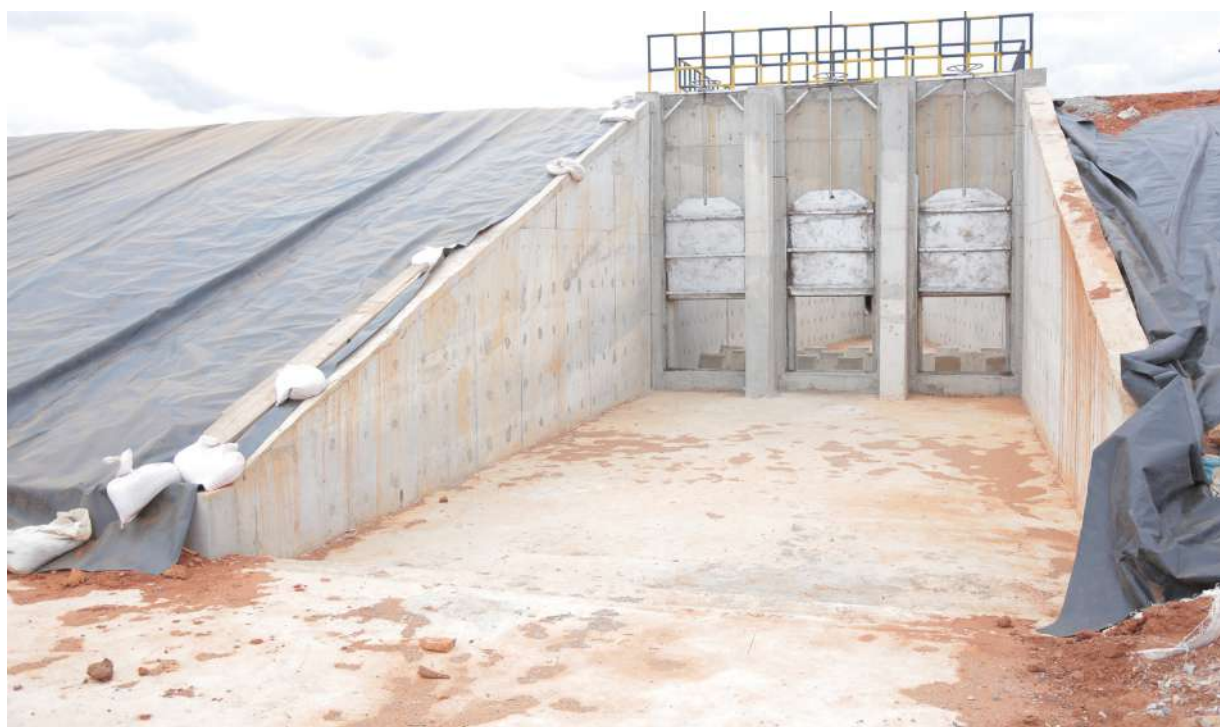
Construction of Irrigation infrastructure in Galana Food Security Project in Kilifi/Tana River Counties
