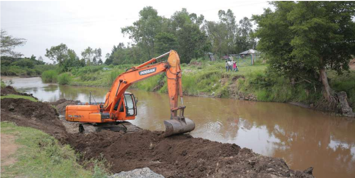
Disilting of a canal in Bunyala Irrigation Scheme
