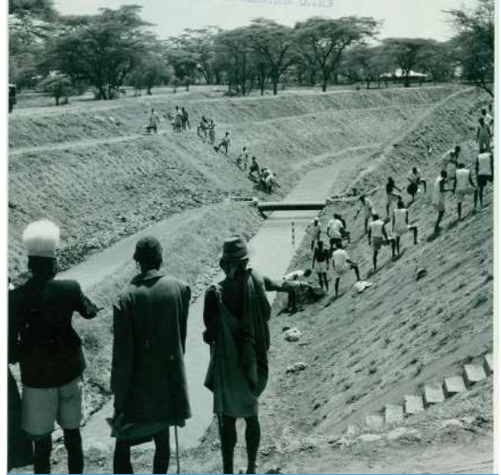
Ilchamus community members study the progress of the scheme's main canal under construction in 1956.
