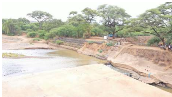
Perkerra Irrigation Scheme Intake.
