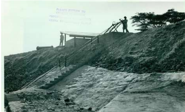
Perkerra Irrigation Scheme canal intake at the boulder weir in 1956
