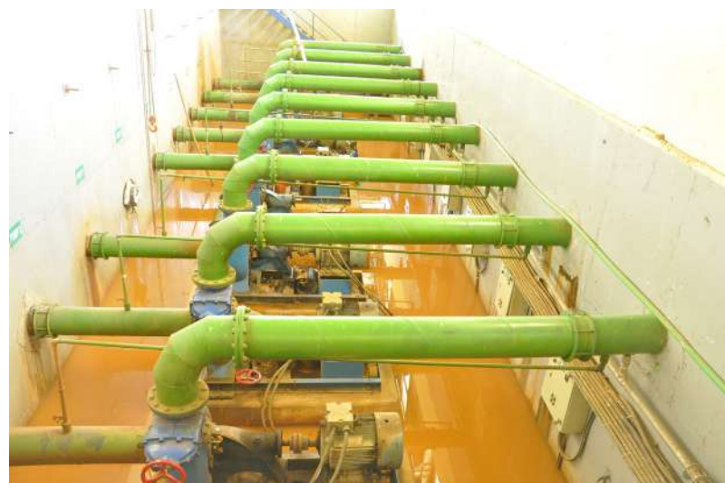
Water intake for Tana Irrigation Scheme
