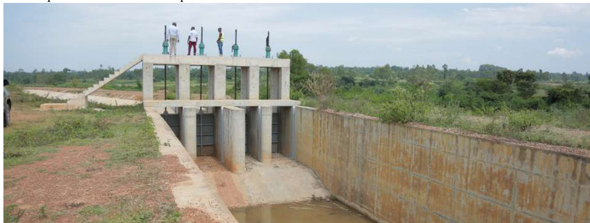
Lined canal in Lower Nzoia Irrigation Project
