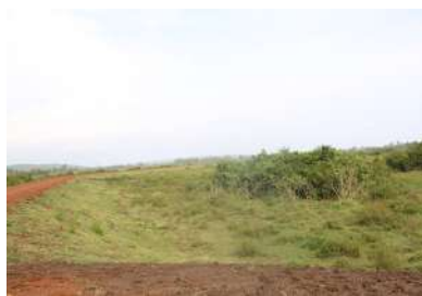
A dyke in Bunyala Irrigation Scheme
