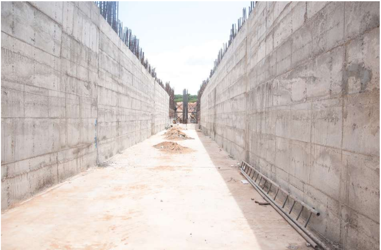
The construction of Bura Irrigation and Settlement Scheme Rehabilitation Project in Tana River County.
