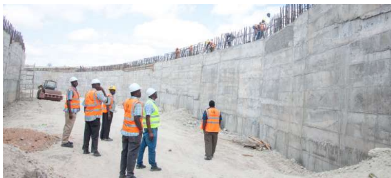
Eng. Joseph Karangu (in green reflector jacket) inspects the construction of Bura Irrigation and Settlement Scheme Rehabilitation Project in Tana River County.
