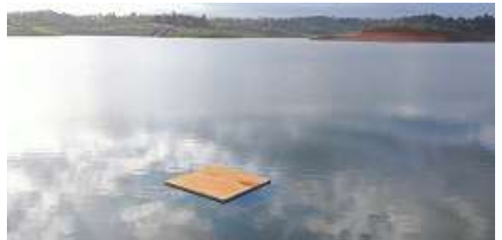
The inlet tower almost submerged in water.
