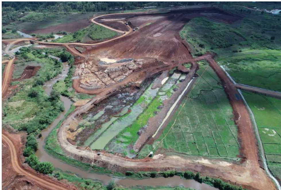
Thiba Dam in Kirinyaga County during its initial construction stages
