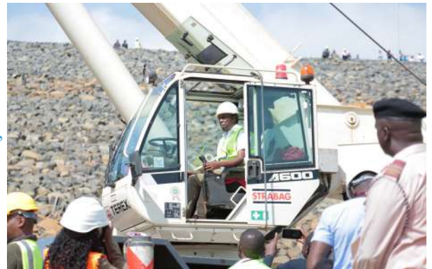
Right; Mr. Gitonga Mugambi EBS, NIA CEO operates a crane to lower Thiba dam's gate.
