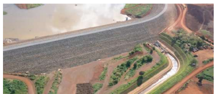
A canal conveying the impounded water to farms for irrigation.
