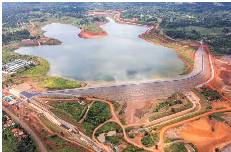
Aerial view of completed Thiba dam in Kirinyaga county
