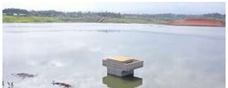
Water levels nearly reaching the top of inlet tower
