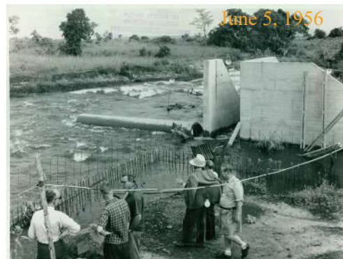
Flooded intake works.
