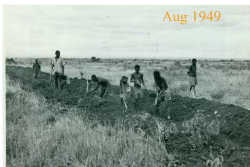
Workmen digging small furrows which was to carry water to the test plots in the pilot scheme.
