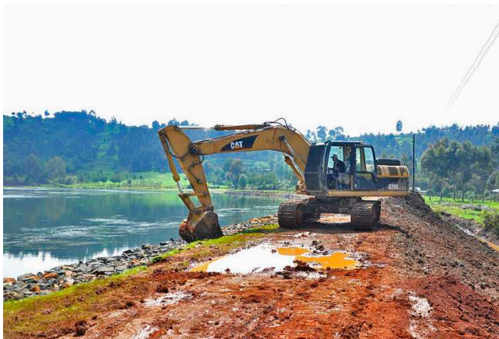
Expansion works in Gwa Kiong'o dam
