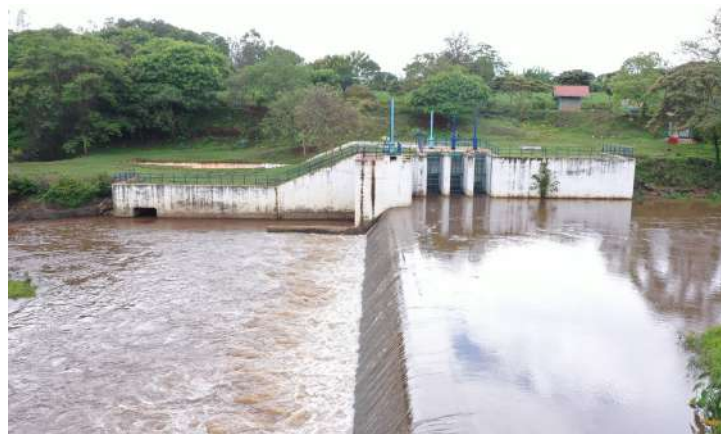
Mwea Irrigation Scheme intake along river Nyamindi
