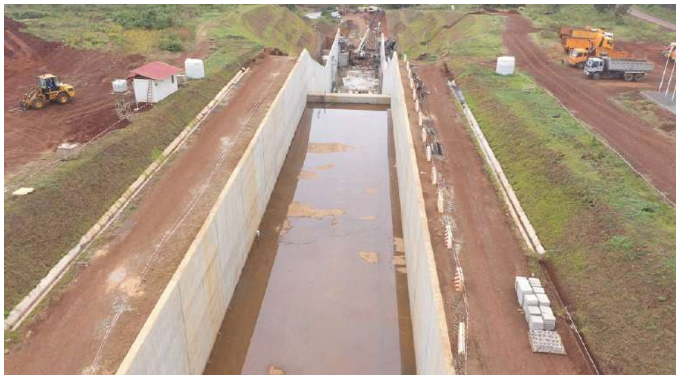
A section of Thiba Dam under construction in Kirinyaga County
