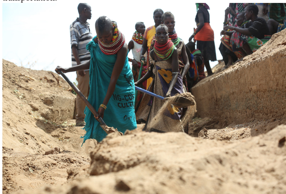
Farmers disilting a canal in Katilu Irrigation Scheme Turkana County
