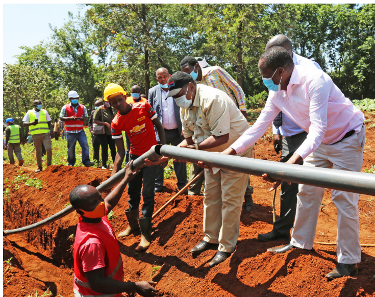
National Irrigation Authority CEO Mr. Gitonga Mugambi(R) with Principal Secretary, Ministry of Water, Sanitation and Irrigation (MoWSI) Joseph W. Irungu, CBS ( center, in black cap) laying a water pipe in Mirira Irrigation Project Murang'a County
