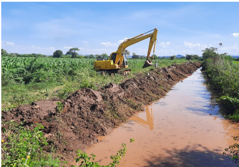
Excavator removing accumulated silt from a canal in Perkerra Irrigation Scheme
