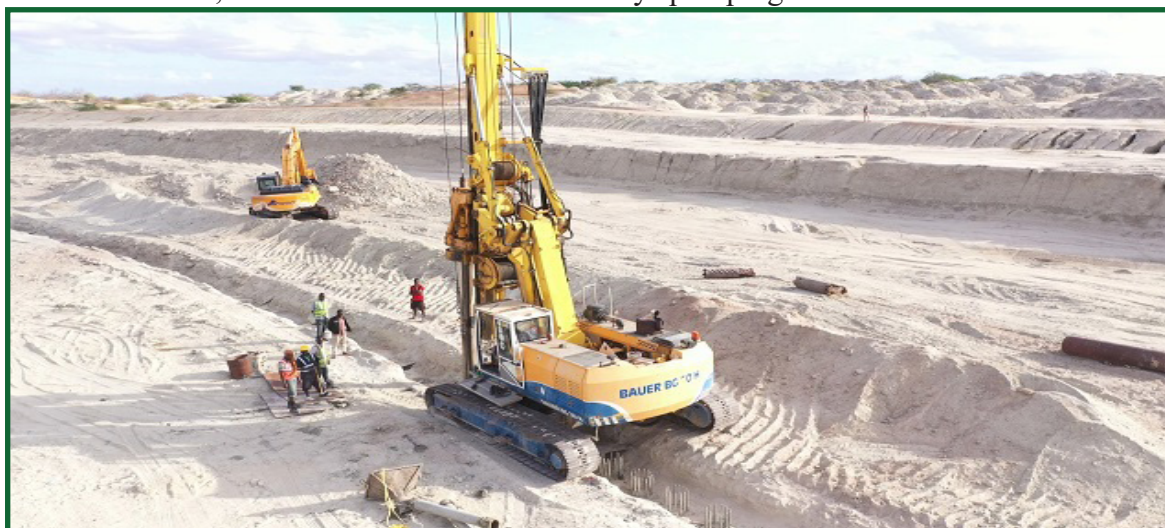
Construction of Gravity fed irrigation system in Bura irrigation development project, Tana River County.
