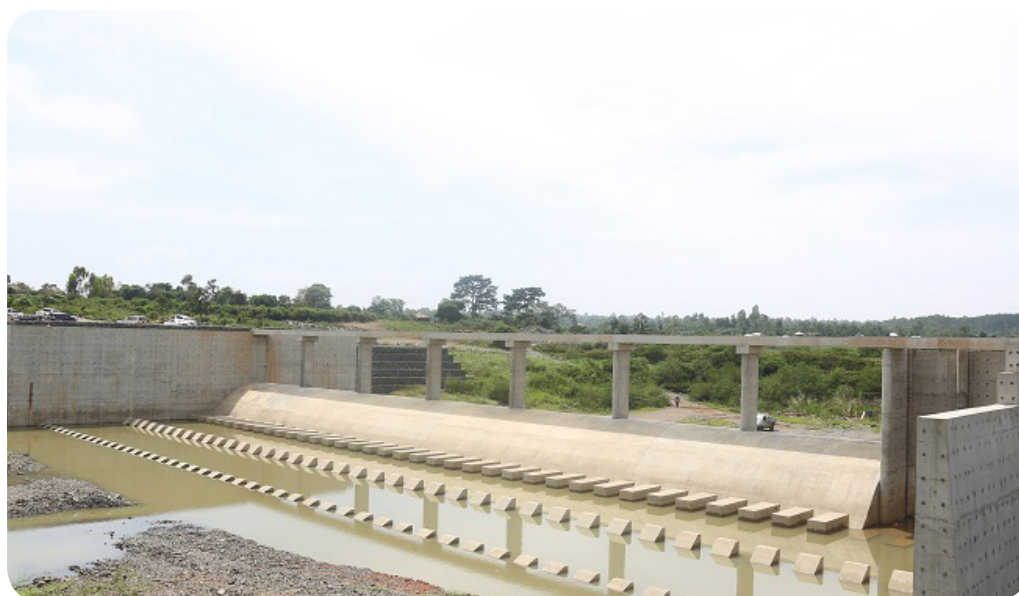
Ongoing Construction of an intake weir in Lower Nzoia Irrigation Project.
